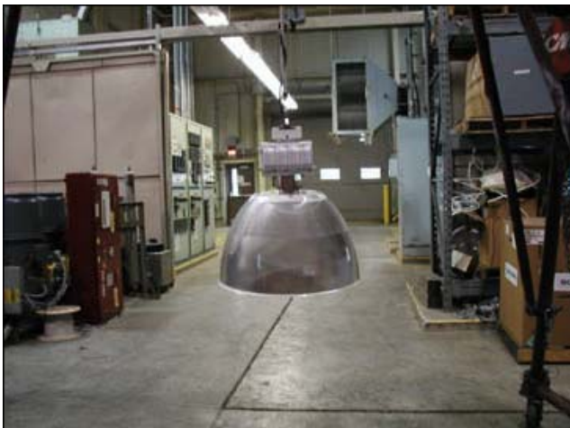
Old Style Lighting Fixture 368 Watts
